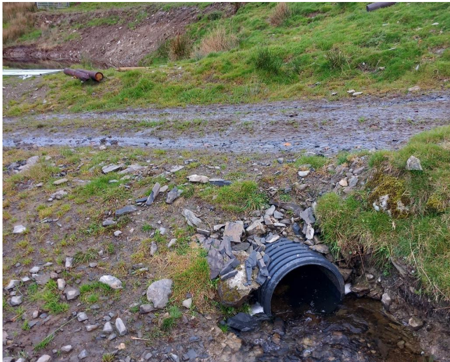
Photograph 7.1.7: Pooled surface water and culvert outlet feeding an unnamed watercourse. NGR SH 92166 41022.
