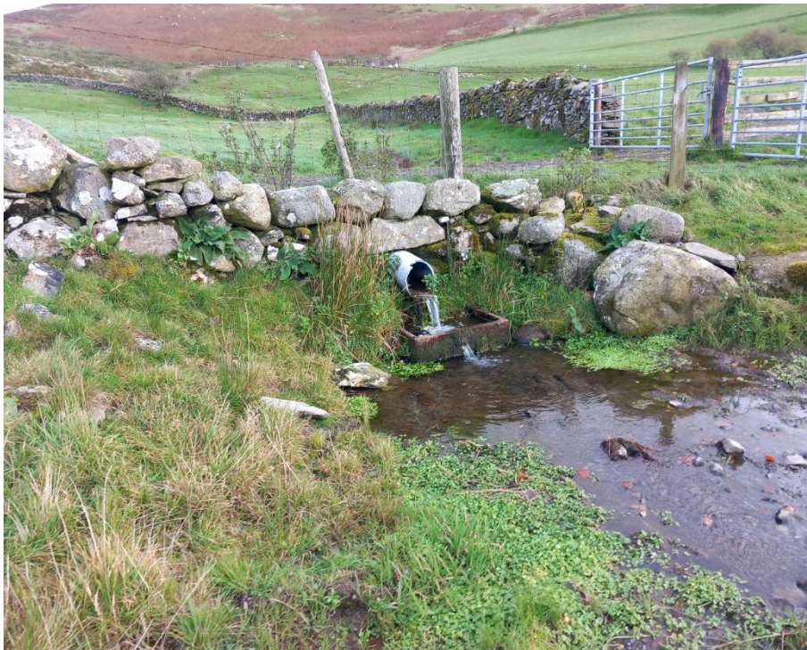
Photograph 7.1.6: Outlet of a culvert diverting a small watercourse under a track. NGR SH 92145 40933.
