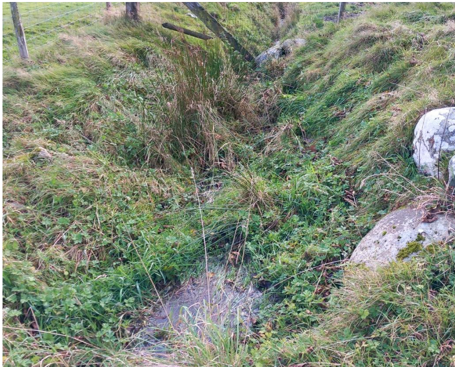
Photograph 7.1.5: Vegetated drainage ditch in poor condition. NGR SH 91841 40884.
