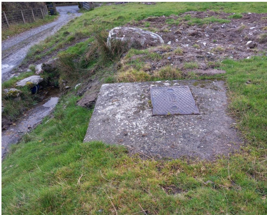
Photograph 7.1.4: Artificial drainage into an unnamed tributary of Afon Mynach. Manhole in the foreground is a disused well. NGR SH 91096 40898.
