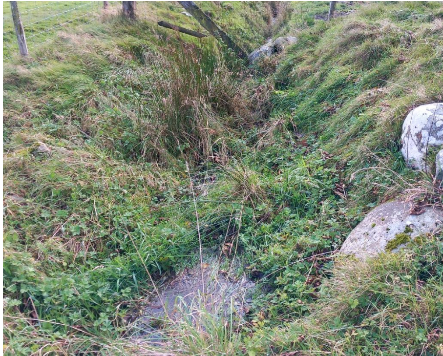
Photograph 7.10.5 Vegetated drainage ditch in poor condition. NGR SH 91841 40884.
