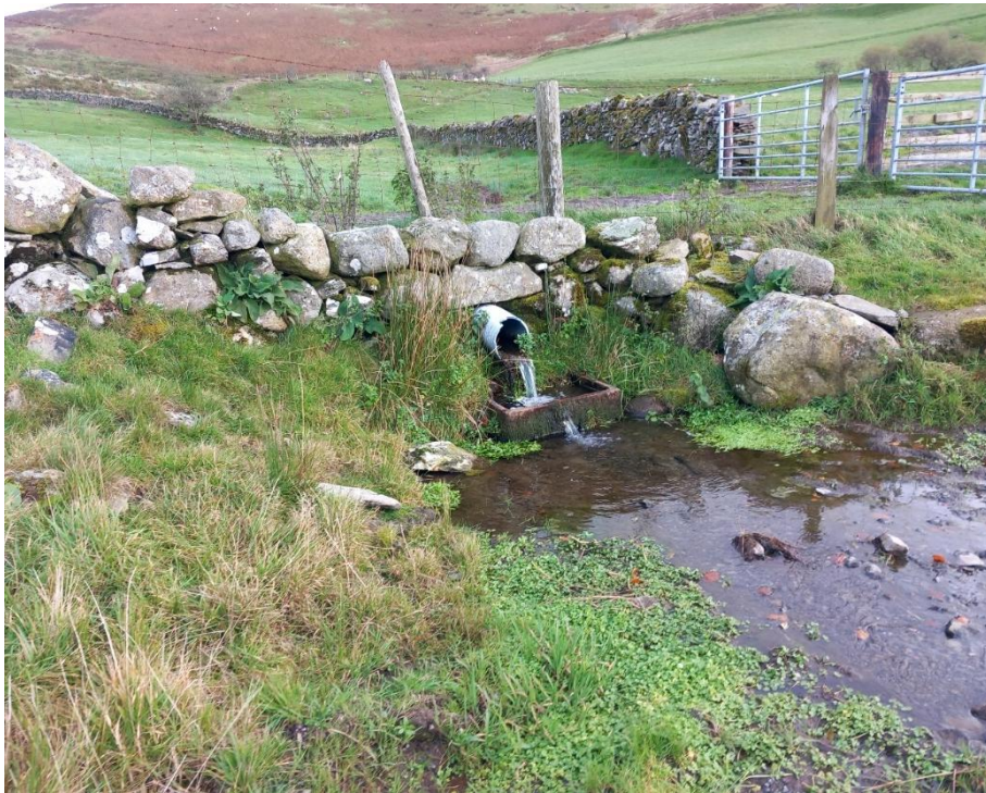
Photograph 7.10.6 Outlet of a culvert diverting a small watercourse under a track. NGR SH 92145 40933.
