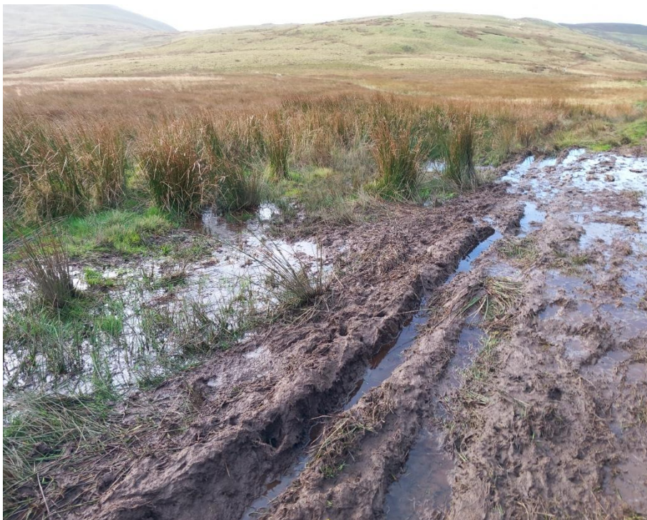
Photograph 7.10.10 Boggy area and Surface water pooling on track. NGR SH 93722 41906
