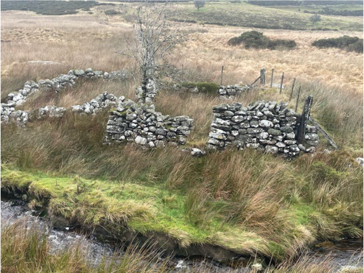
Photograph 12: Dilapidated sheep pens boundary of RLP1 and CL59
